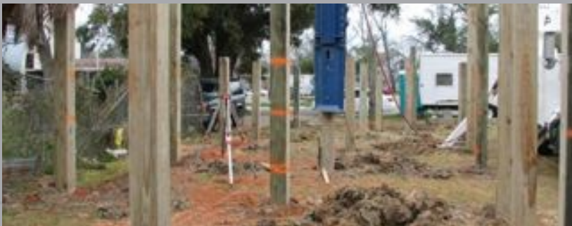
Robinson home, driven wood pile foundation detail. [Diagrams not to scale.]
